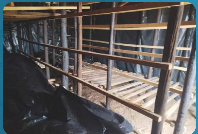
Fig 6: Mushroom house design showing the plastic lining on the walls and shelving of the growing room to accommodate multiple production system
